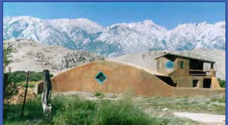
Anchor Ranch House, Lone Pine, California This was the first permitted straw bale building in California
